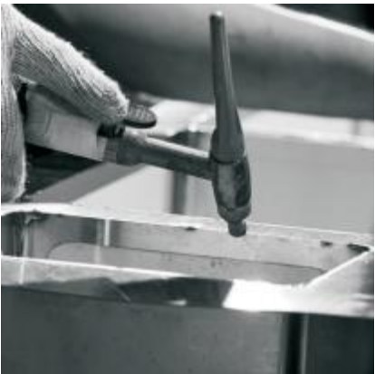
7 STRUCTURE SPLICING FOR PANEL&SINK
